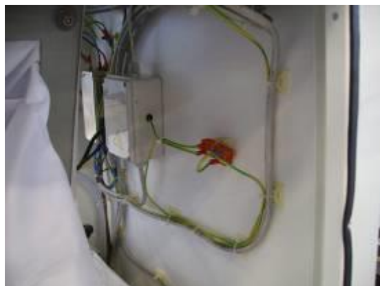
Earth connection during the maintenance operation
